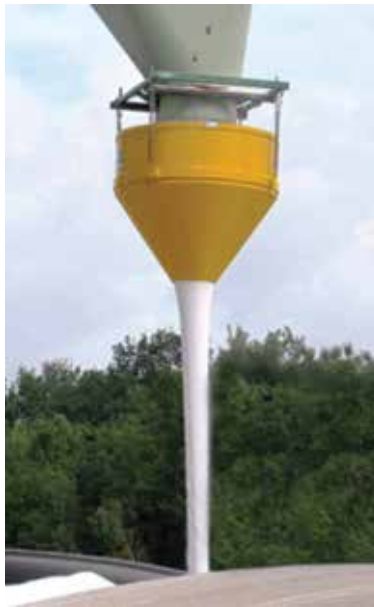
FIG. 2. Dust suppression hopper (dustless spout) from Sioux Steel Company
